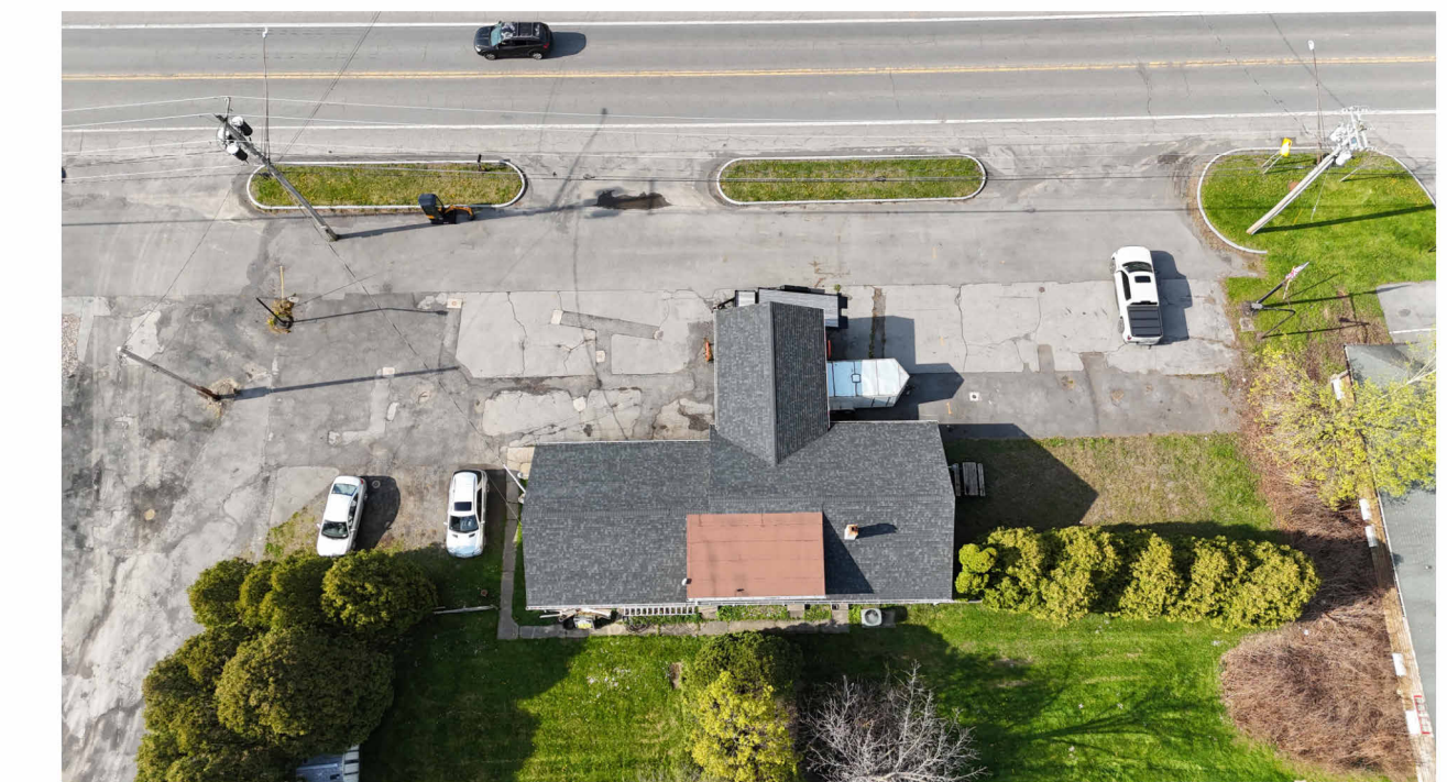
7 Existing Conditions - Roof View
