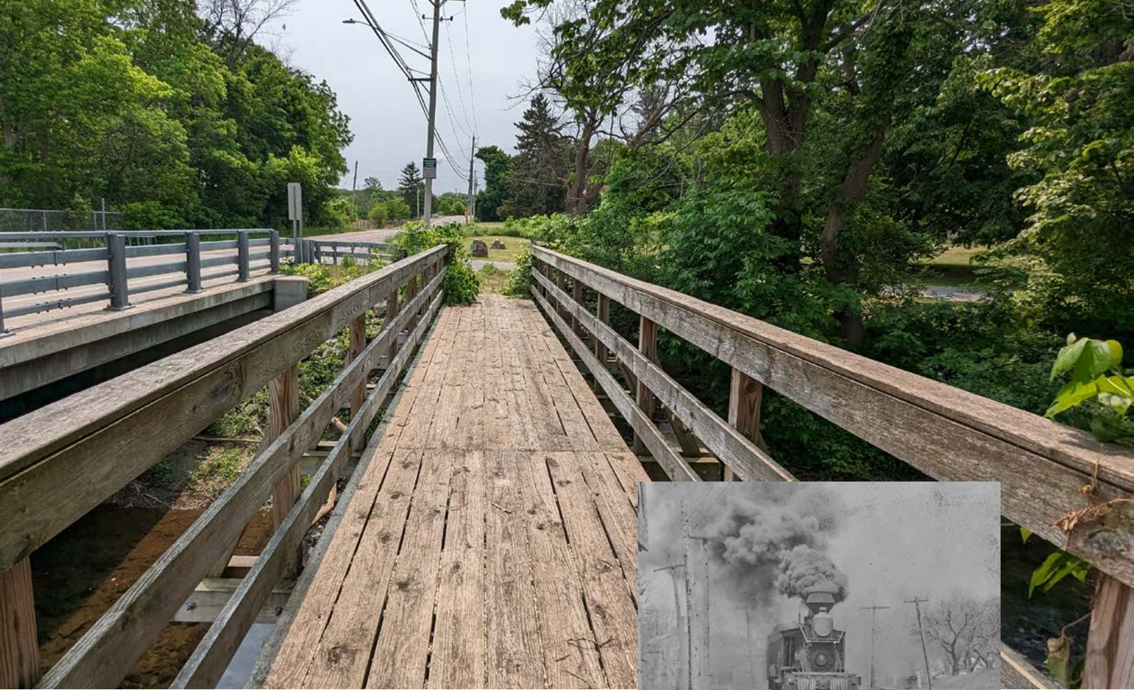
Pedestrian Bridge over Skaneateles Creek on former railroad bed
