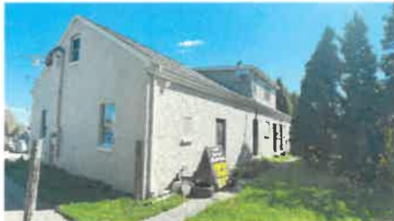
2 Existing Building Elevation - North
