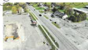
29 Existing Conditions - South View
