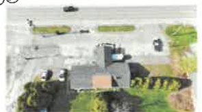
30 Existing Conditions - Roof View
