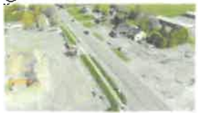
Existing Conditions - South view
