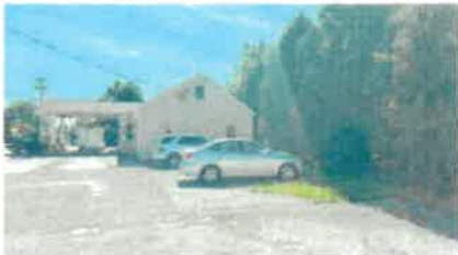
13 Existing Building Elevation - East
