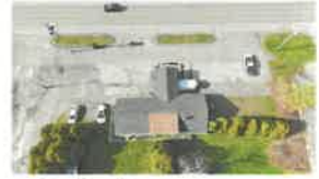
7 Existing Conditions - Roof View
