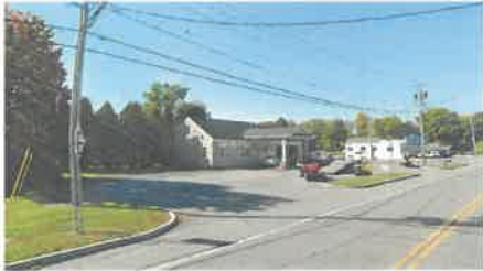
24 Existing Building Elevation - West
