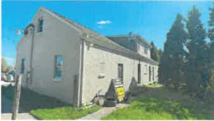
28 Existing Building Elevation - North
