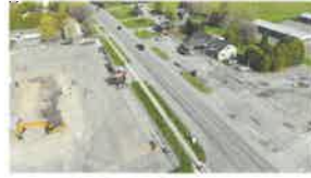
6 Existing Conditions - South View
