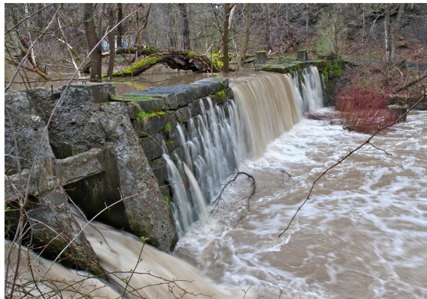
Dam, Skaneateles Creek
